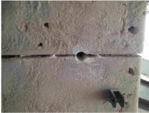
'Keyhole Surgery' is used to make Electrical Connections (Left). Anode Mesh Installation (Right)
