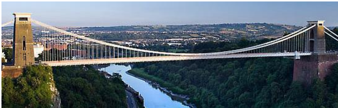
Clifton Suspension Bridge – Based on Designs by Isambard Kingdom Brunel
