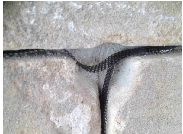
'Keyhole Surgery' is used to make Electrical Connections (Left). Anode Mesh Installation (Right)
