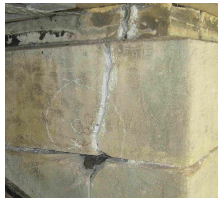
Both Lifting of Stonework (Left) and Cracking (Right) are the Result of Corroding Embedded Ironwork
