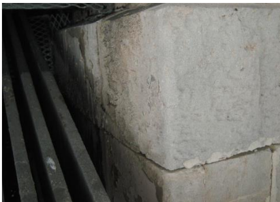
Both Lifting of Stonework (Left) and Cracking (Right) are the Result of Corroding Embedded Ironwork
