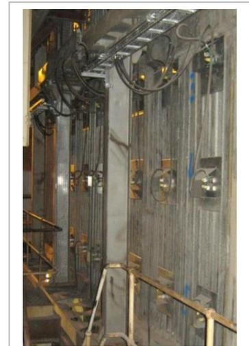
*Scanner Sensor Array: Boiler Membrane Wall*
