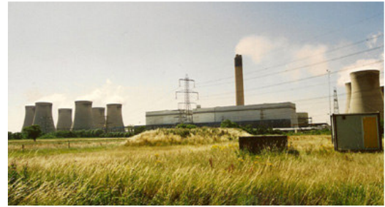
Drax Power Station, UK
