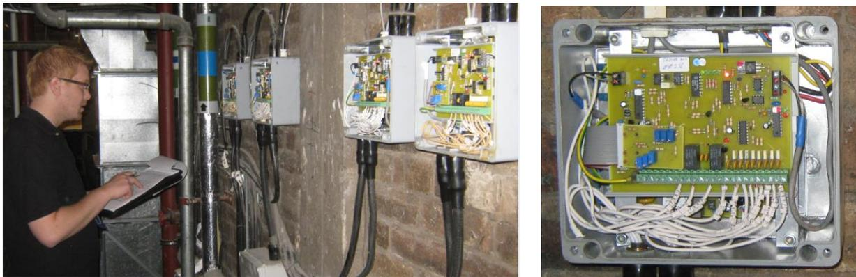
New LRU Circuit Boards installed within Existing Enclosures with Adequate Room for Wiring
