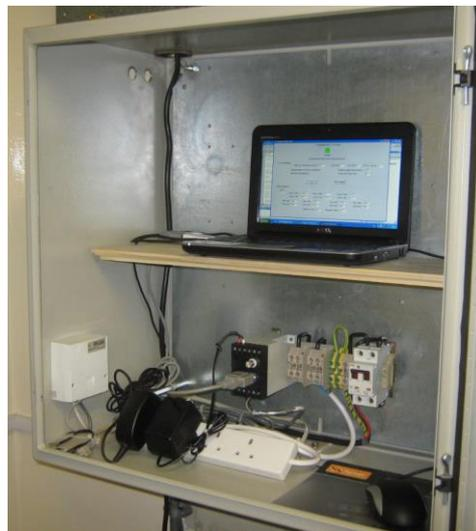
The Main Cabinet was also Refurbished: a New Data Logger was Installed together with an ADSL Link for Remote Communications
